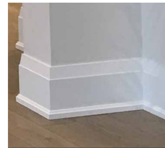
Contemporary interior trim package (4" baseboard and 2-3/4" casing).
