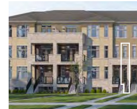
FRONT, Interior Unit
